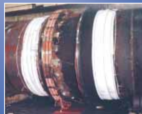
In-shop stress relieving of kiln weldments.
