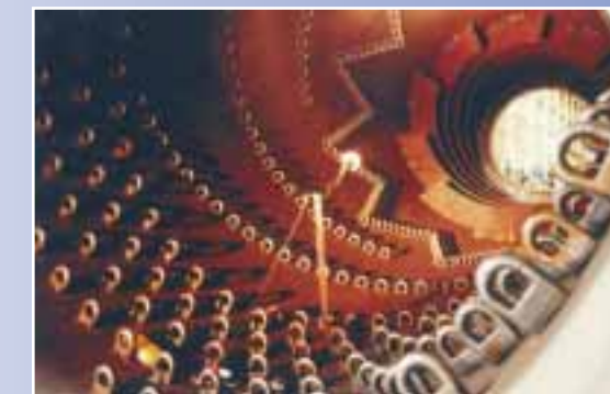
Internal fittings of rotary kiln for Pulp and Paper Mill.
